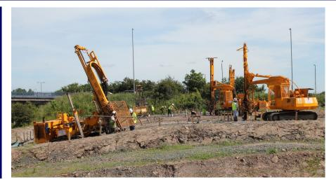
Advance Groundworks contract to consolidate worked coal seams and overburden at a) the site of Scottish Gas Networks (SGN) proposed new TRS and b) on the proposed line of diverted high pressure gas mains. SGN will construct the TRS and the gas main diversions prior to the main M8 M73 M74 Motorway Improvements contract. The works were located south of the A8 at the Shawhead Junction (A8/A725), Coatbridge as shown.
